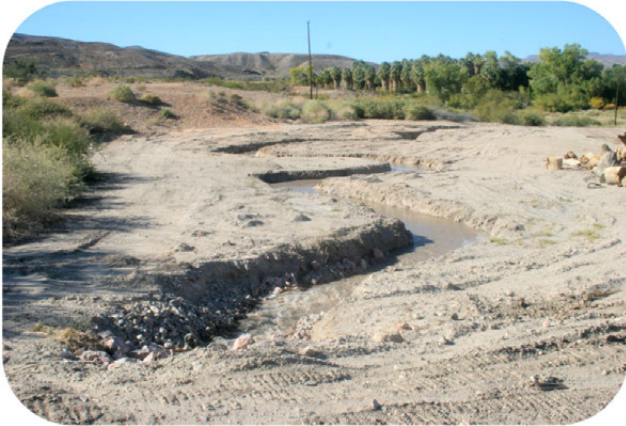
Pederson Channel construction © David Syzdek
